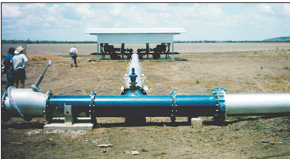
Part of the work for this project, at the property of Bill Cragg, Dingo, was conducted by Greg Cross.
